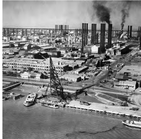
The AIOC oil refinery at Abadan in 1951.
